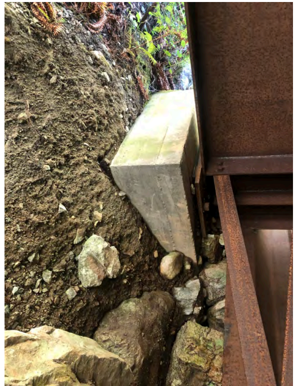
Left Bank Abutment when facing downstream
