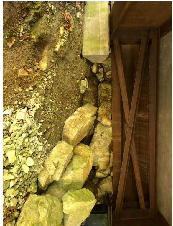
Left Bank Abutment when facing downstream
